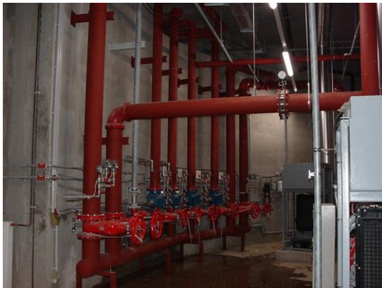
sprinkler water distribution system
