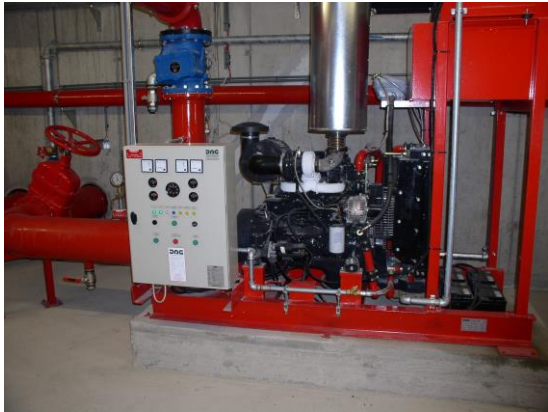
diesel driven sprinkler pump
