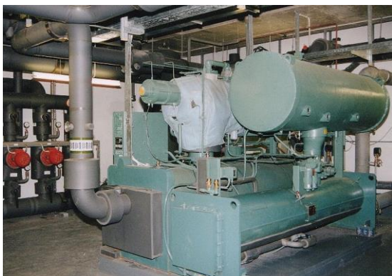
5 nos water cooled chiller total cooling capacity 5.000 kW
