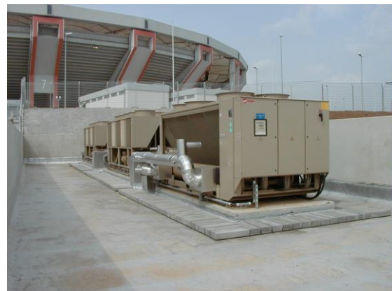
3 air cooled water chillers on roof of technical building total cooling capacity: 2.000 kW
