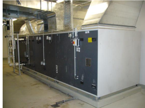
total supply air volume 1.008.900 m 3 /h (58 air handling units)
