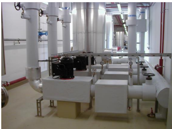
chilled water pipe work with pumps in technical building
