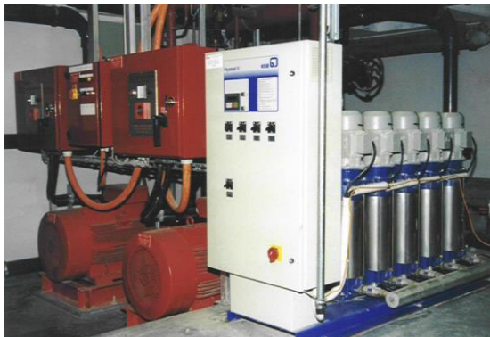
sprinkler pumps and potable water booster station (7.000 sprinkler heads, 40 fire hydrant cabinets)
