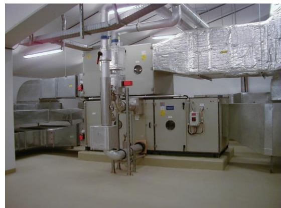
one of nine air handling units in two plant rooms
