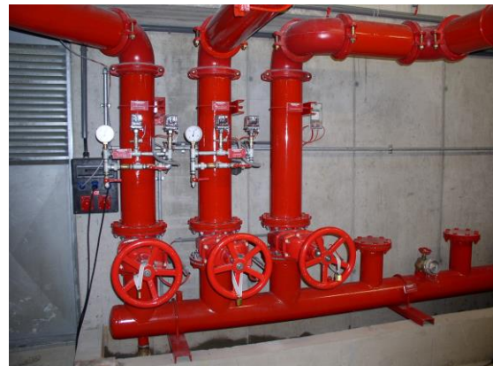
sprinkler valve station
