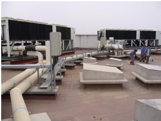
total chilled water capacity: 6.800 kW (8 chillers with 850 kW each)
