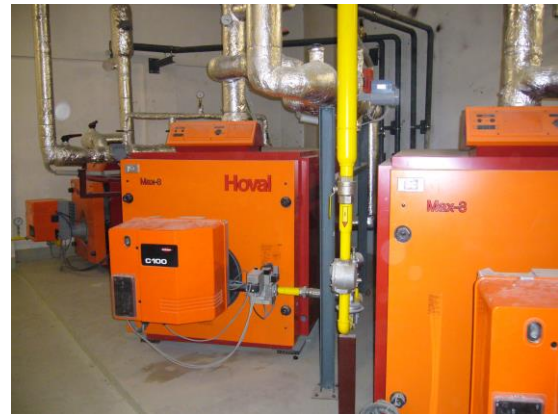
total heating capacity: 3.120 kW (4 boilers with 700 kW each, 1 boiler with 320 kW)
