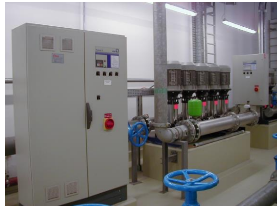
booster pump sets for hydrant water system (for 80 fire hydrant cabinets with hose reels)
