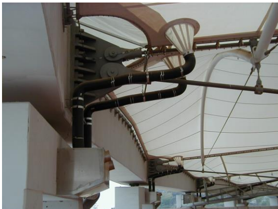
drainage of stadium roof
