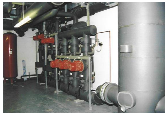
chilled water distribution pumps
