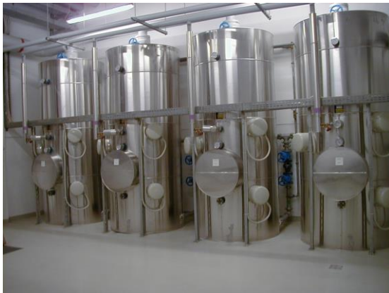
hot water production with four electrical water heaters
