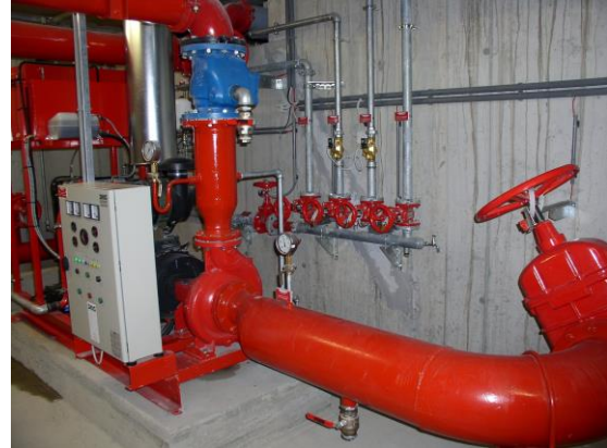
electrical driven sprinkler pump
