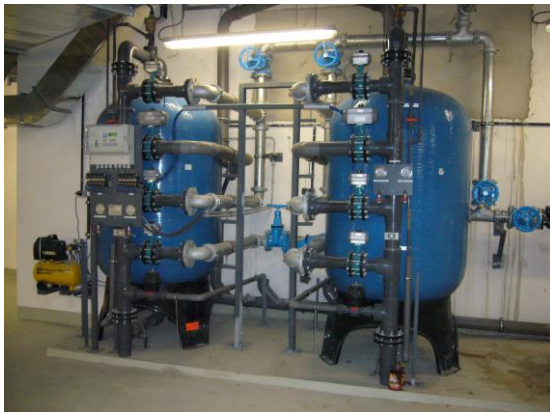
part of water treatment (for a water volume of 76 m 3 /h)
